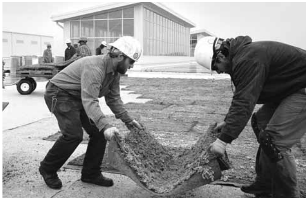
Workers install the Living Roof at the Rouge Center.
